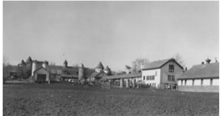
The dairy barns, built in 1915, are in the background and to the right are sheds for cows, calves and bulls. The two story structure used by the Animal Nutrition Department and the veterinary hospital is to the far right.
