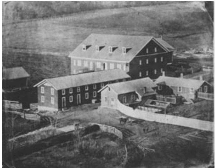
After Old Main was completed, the shacks were removed. This barn and out buildings were lost to fire in 1897.
