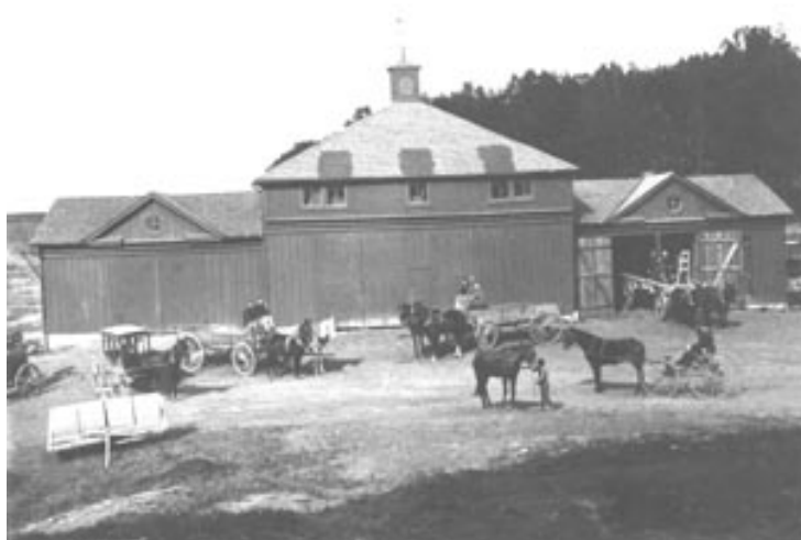
New West Barns, built 1897-98, were located below Rec Hall at the intersection of Pollack Road and Atherton Street
